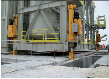
Fig. 1 - Drilling mud tank handling
